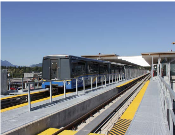
Testing and Commissioning at Burquitlam Station
