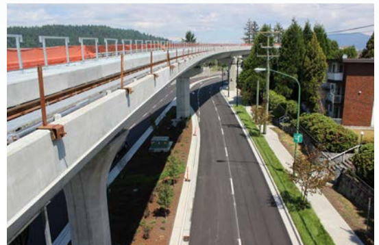
Guideway and road improvements on North Road
