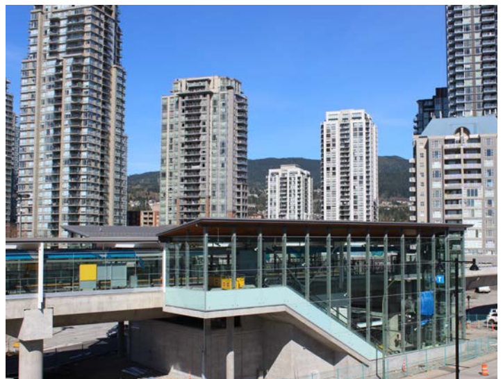
Lincoln Station in Coquitlam
