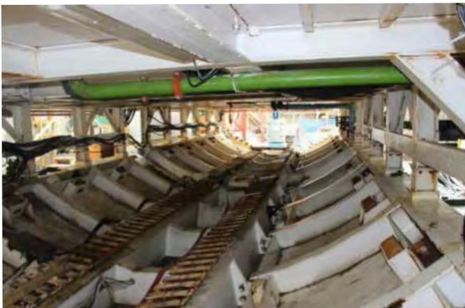
*The ring segment conveyor delivers precast segments to the ring erector.*
