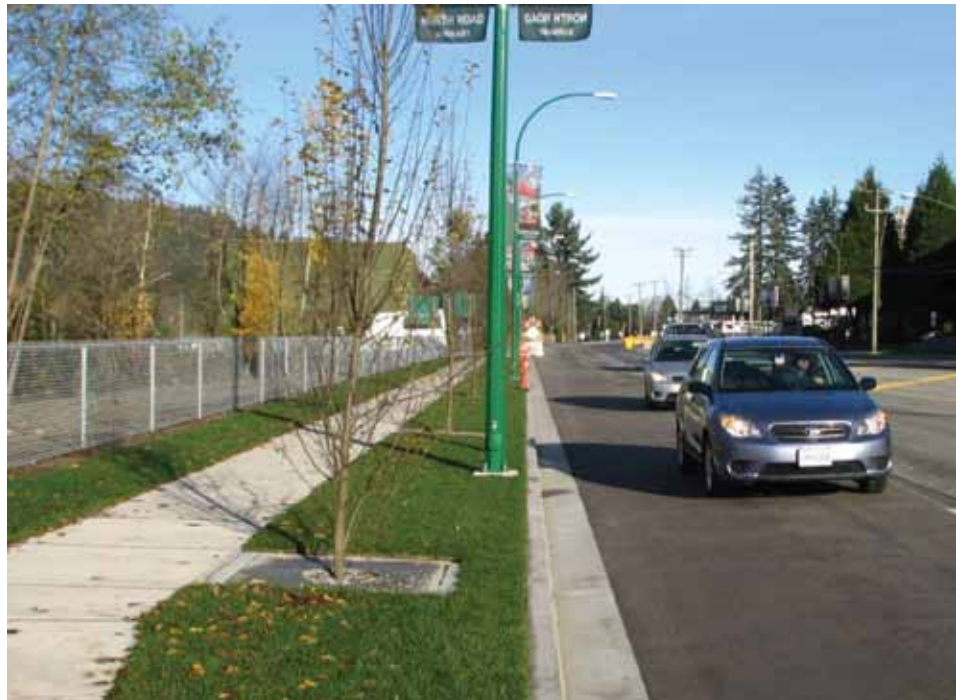
Boulevard-style sidewalks and street trees on the west side of North Road are some of the aesthetic improvements included in the North Road widening project
